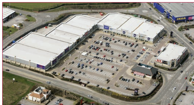
Junction 27, Birstall, Leeds
