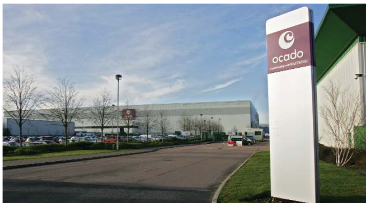
Ocado Distribution Unit, Hatfield
