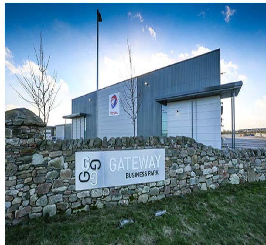
Completed Total building at Aberdeen Gateway
